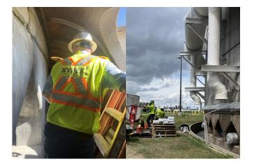
The solution came in the form of Xypex MegaMix II with Bio-San, which is a cement-based resurface repair mortar designed for use in harsh environments.
